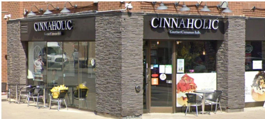
Figure 4-3: Use of Masonry on Building Façade (Brick and Stone)
